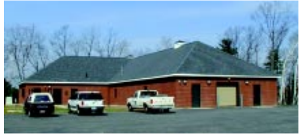
LWD's Spectacle Pond Treatment Facility
