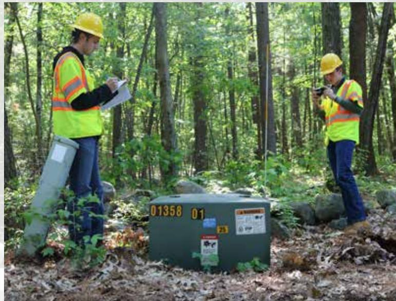
Electrical interns Tyler Hunt (left) and Joe LeDuc (right) inspect a padmount transformer as part of their work this summer to identify parts of the system in need of maintenance which helps to prevent outages.
