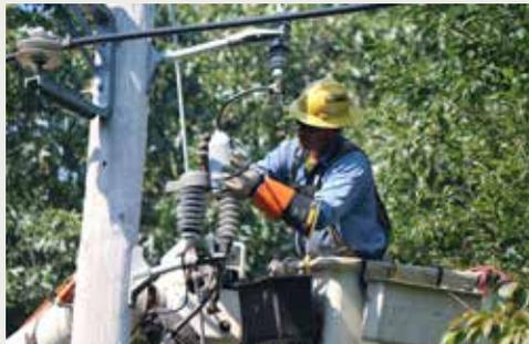
*LELWD’s award for reliable service is in part due to the proactive maintenance on the system. The installation of squirrel guards on the system has sharply reduced the number of outages due to wildlife. Lineman Todd Burnham installs a squirrel guard on Whitcomb Ave.*
