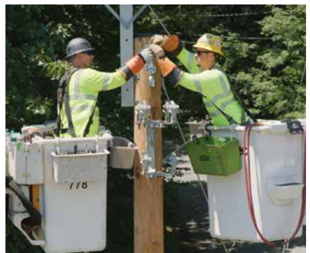
Equipment to keep line workers safe includes hard hats, arc-rated clothing, harnesses, insulated gloves and eye protection.
